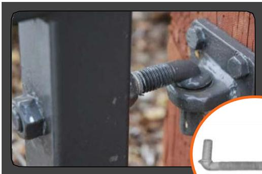
J-bolt hinge connects post to the wall
