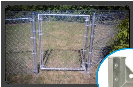
Gate corner uses for attaching gate corners
