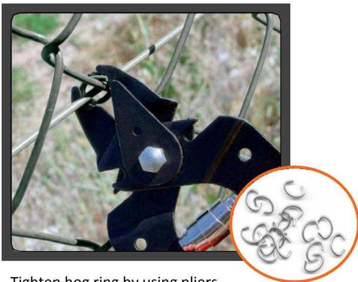
Tighten hog ring by using pliers
