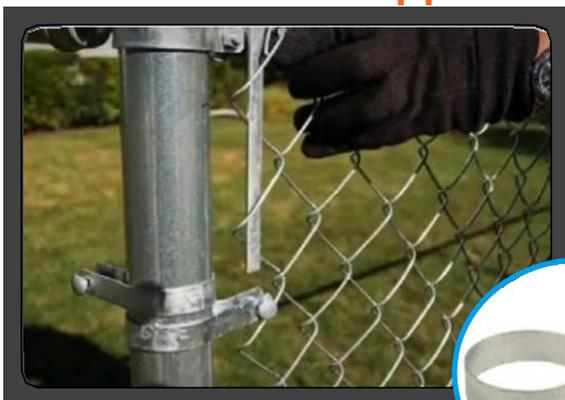
Tension band reinforces chain link fence
